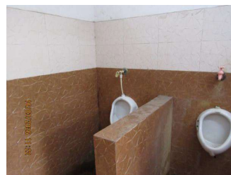
NC - No water connection pipe in urinals.JPG
